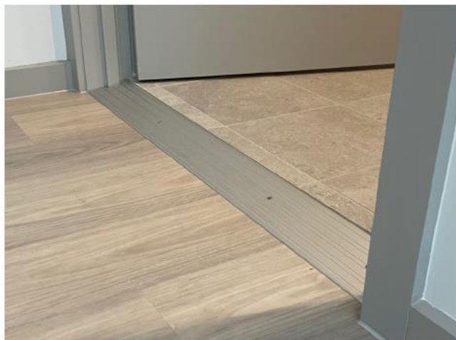
Figure 12 - Example of a ramped threshold within a door jamb
